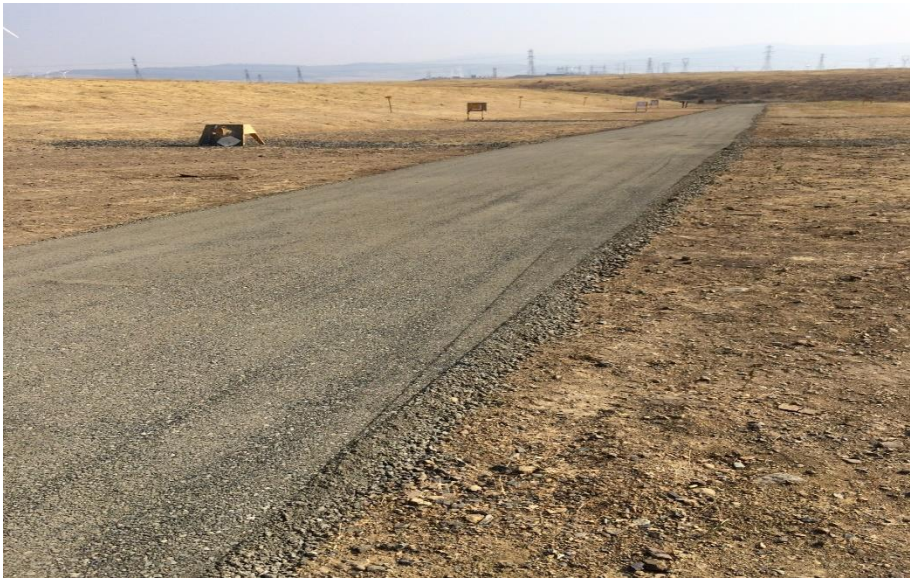
New 8 foot wide pathway ready for asphalt on Rifle Range.
