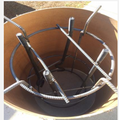
Sonotube and rebar forms.
