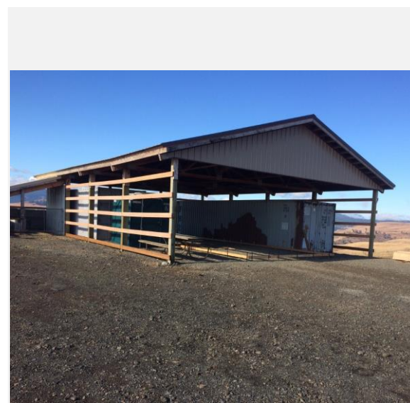
Ready for metal siding
