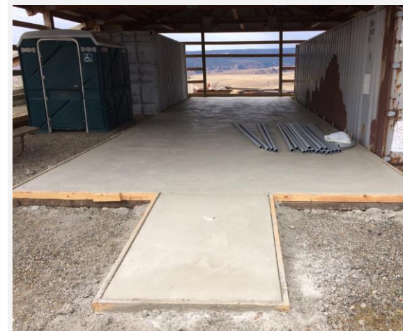
Floor for future meeting room
