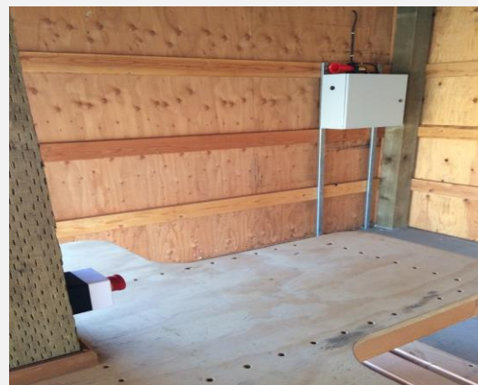
Cease fire alarm system is up and running. Read instructions on post.
