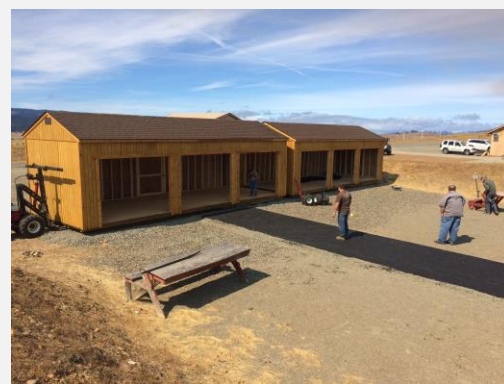
New pistol range sheds being set up
